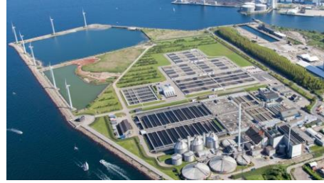
1998 New sewerage treatment facility constructed
